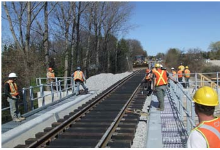
New Unionville GO train bridge completed
