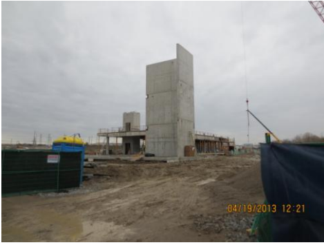
Pan Am Centre is under construction.
